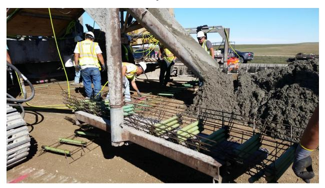
The base was reworked on the project and gravel pre-trimmed, but left a little high. The "lowa Special" unloading machine also performs the final trim of the base course cushion material leaving a fresh uniform cross section and base for the new concrete surfacing.
