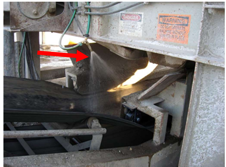
Photo: Dwayne Stenlund, MnDOT
