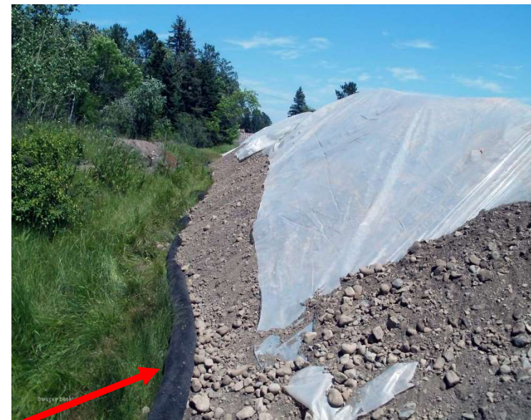
Plastic cover and perimeter berm
