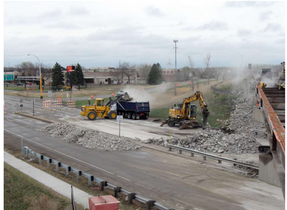
Photo: Dwayne Stenlund, MnDOT
