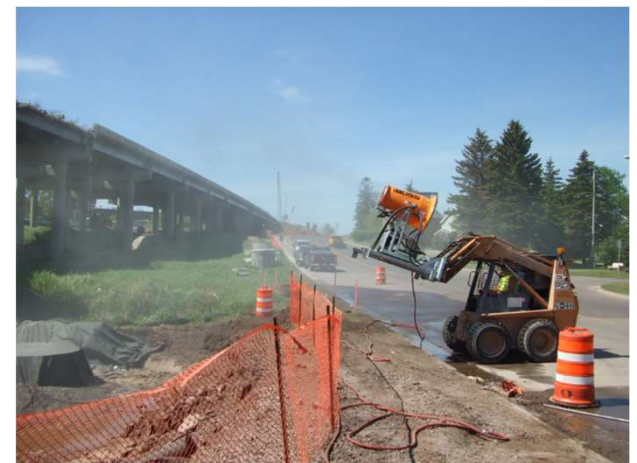
Photos: Dwayne Stenlund, MnDOT 32
