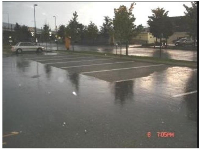
Pervious Concrete Pavement Test Section After Storm Event
