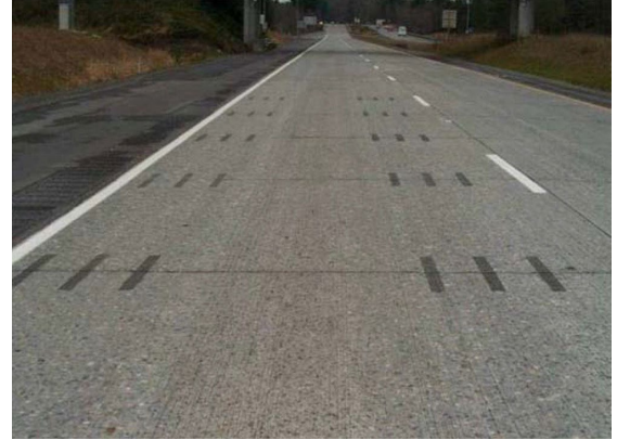
Roadway rehabilitated with LTR & DG
