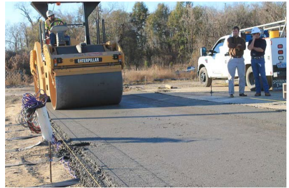
Compaction of RCC
