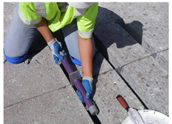
Inserting dowel assembly into slot for dowel bar retrofit
