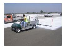
performance-based evaluation of the effectiveness of curing techniques in preventing moisture loss in concrete pavements.
