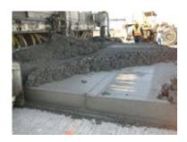
Two-lift concrete paving can be categorized under <u>CP Road Map Track 13: Concrete Pavement Sustainability</u>. It also contributes to <u>Track 4: Optimized Surface Characteristics for Safe, Quiet, and Smooth Concrete Pavements</u> because the top lift can be optimized to meet surface needs such as low noise and friction.
