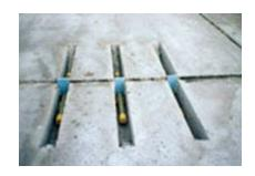
Retrofit Performance in Wisconsin, also suggest that mortar fill material must be mixed, placed, and cured properly in order for DBR techniques to be most efficient.
