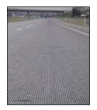
the on-board sound intensity (OBSI) test method, which confirmed a noticeably quieter surface than the previous section. Friction measurements were also very favorable, as expected with a newly ground surface.
