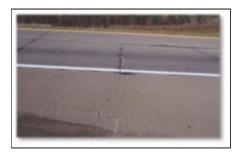
weather conditions can cause pavement distress due to the potential of one pavement to be in tension while the adjacent slab is in compression. To avoid this, care should be taken to avoid paving adjacent lanes during drastically different temperature conditions.
