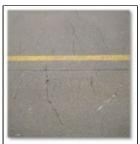
With regards to moisture loss, it was found that the curing compounds with the wax did perform slightly better than the non-AMS resin. An increase in the percent solids from 37 to 44 percent did result in a lower moisture loss for the AMS resin. The benefit of the increase in the percent solids was not as apparent for the wax-based curing compounds. The moisture loss between the wax based curing compounds was very similar.
