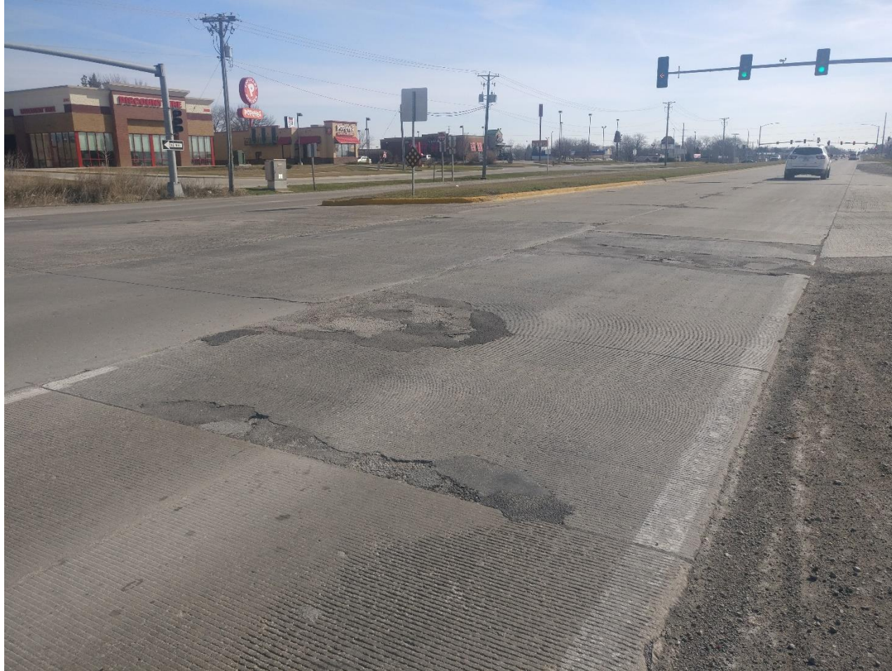
Joint deterioration
