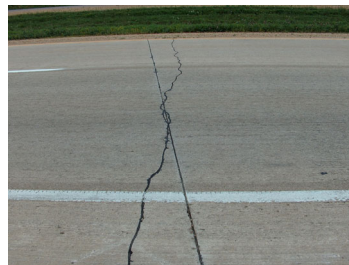
Late sawing crack
