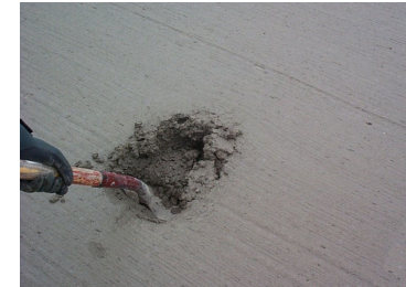
Sampling concrete behind the paver
