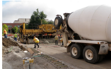
Ready mix truck – 90 minute time limit
