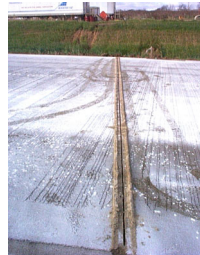
Residue from early entry sawing
