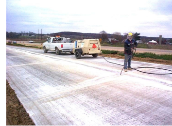
Air blast of joint prior to sealing
