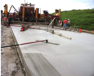
Hand float and straight edge
