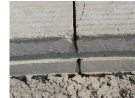
Blowout at edge of slab
