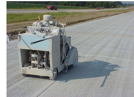
Conventional saw on longitudinal joint
