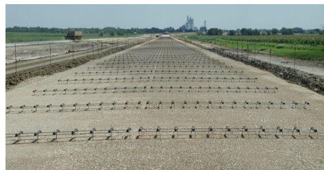
Sighting the grade for dowel alignment
