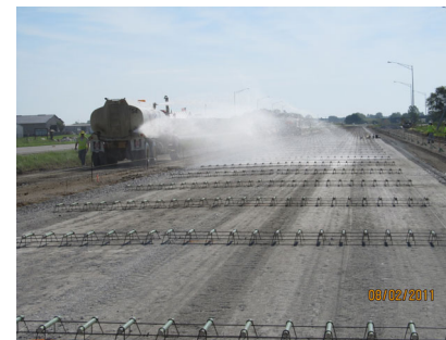
Grade must be moist ahead of the paver
