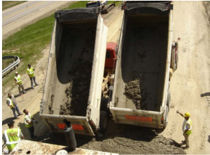
Dump truck – 30 minute time limit May be extended 30 min with approved retarder
