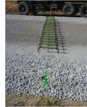
Paint mark to guide sawing operation
