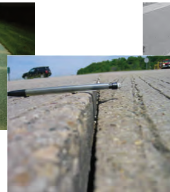
Transverse Joint Faulting
