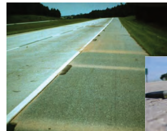
Loss of Fines (Pumping)
