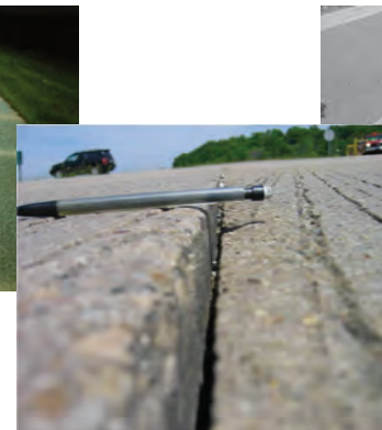
Transverse Joint Faulting
