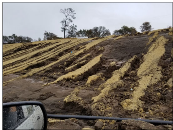
Slope failure due to burnt out HDPE Pipe
