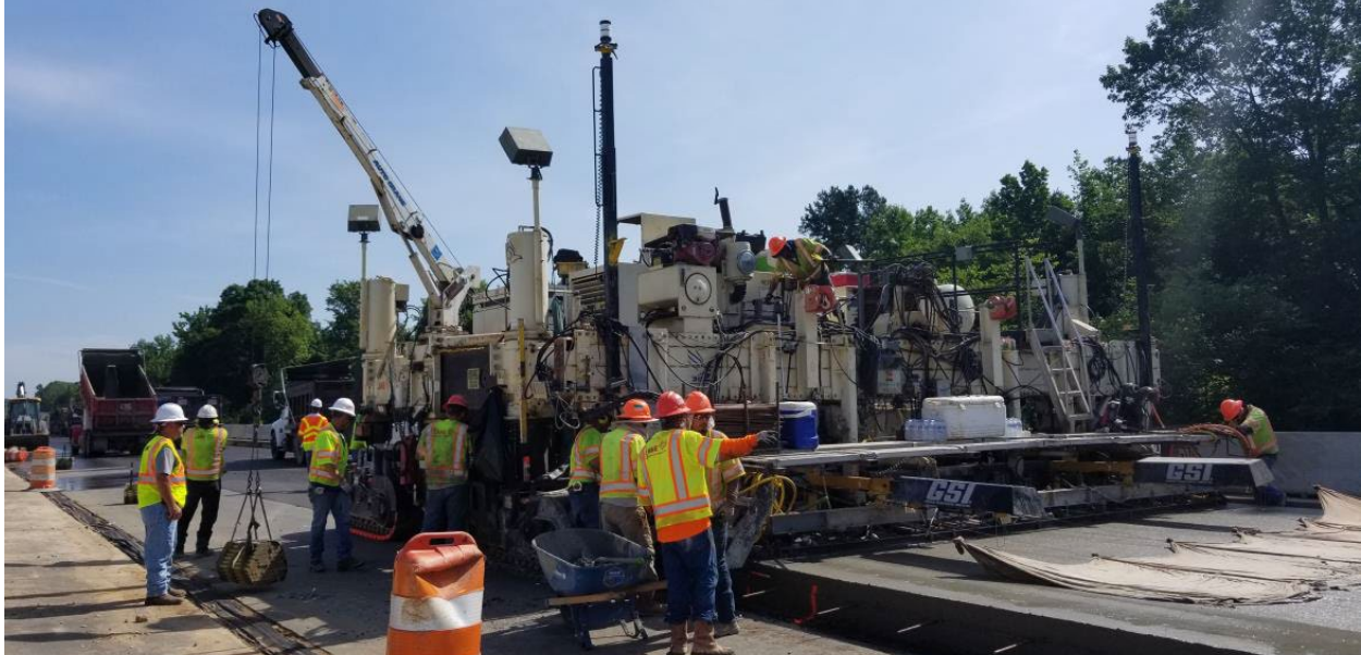
G&Z paver with DBI technology and real-time smoothness measurement used for mainline pavement (source: reference 1 )
