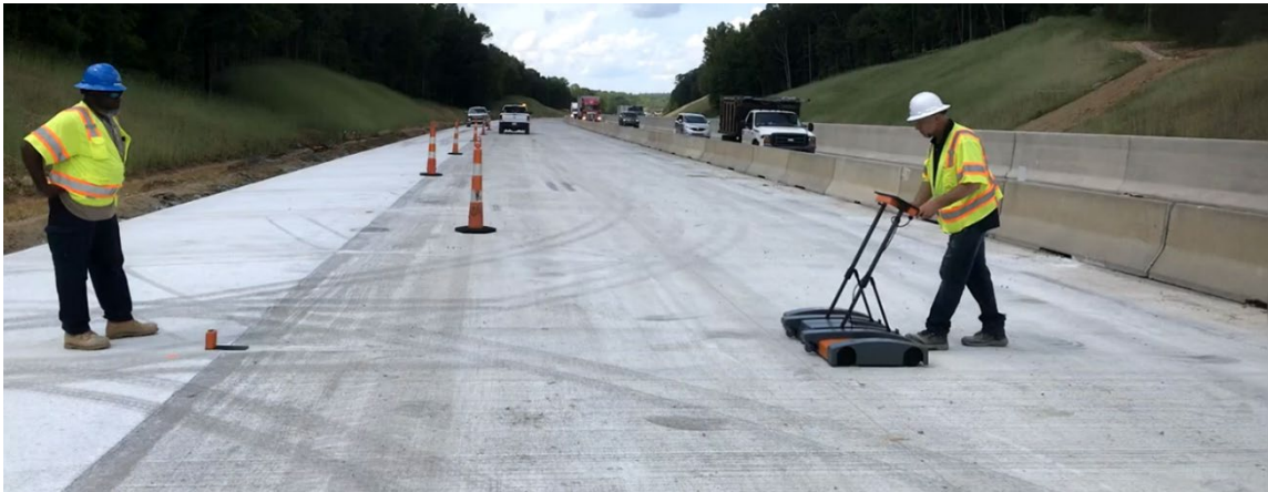
MCTC Personnel using the MIT Dowel Bar Scanner on Mainline Section
