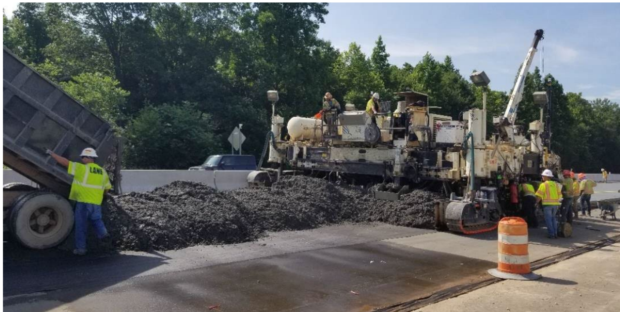
Concrete placed onto asphalt interlayer prior to entering paver (source: reference 1)
