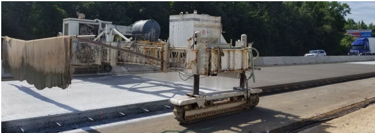
Curing Operations (source: reference 1 )
