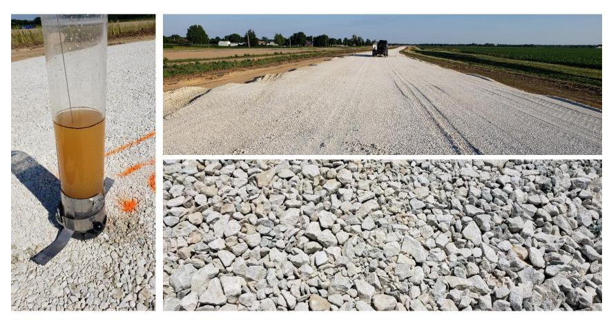
US61, Des Moines County (06/16/2020) Granular Subbase – Crushed Limestone
