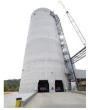
2009-10 Creek Relocation - 26,800 CY Soil Stabilization, Creek Lining, Tunnel Under Plant 2010 New Cement Silo – 5,100 CY Slip Formed – 5100 CY (40% Slag) Intricate Structural Design
