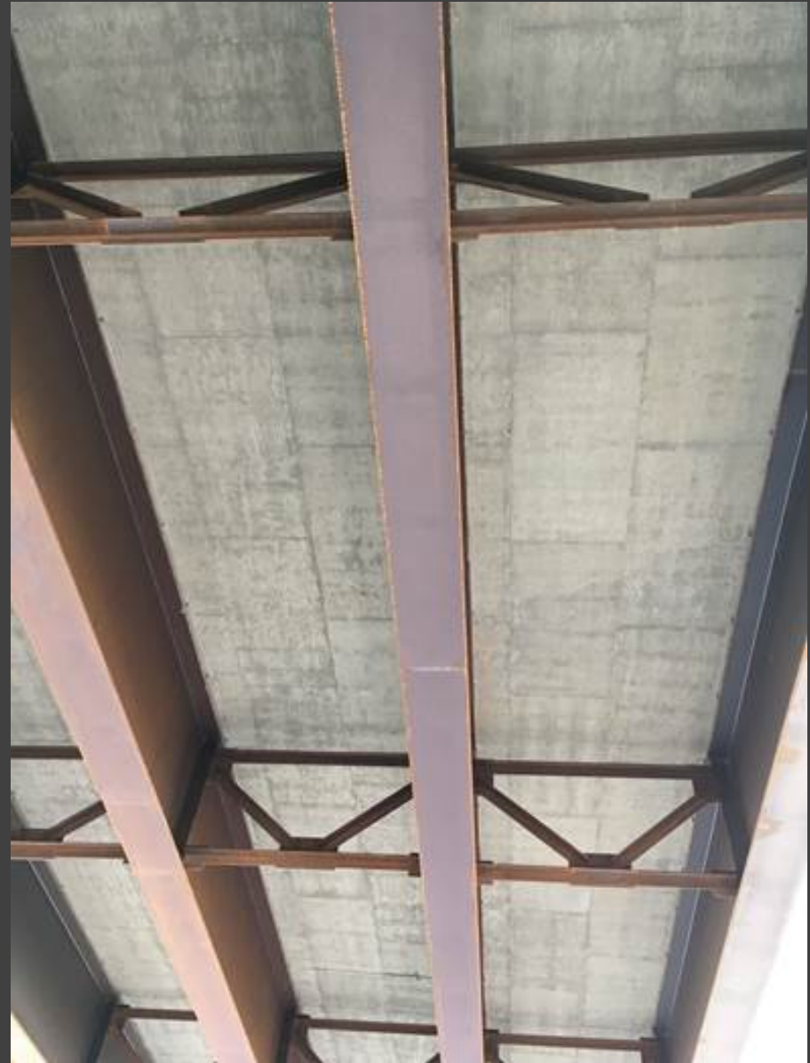
Southbound Structure built 2017
