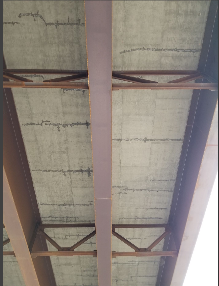
South Bound Structure 2019
