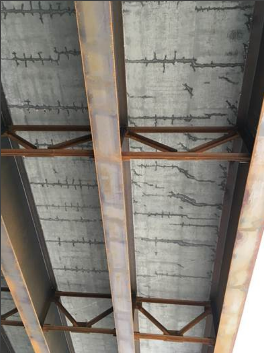
Northbound Structure built 2016
