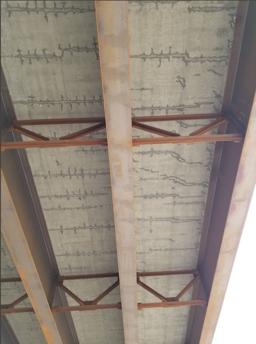
North Bound Structure 2019
