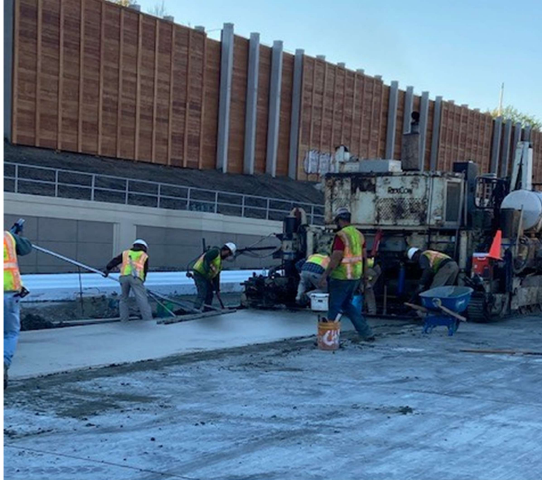
Figure 3. Overview of paving operations.
