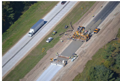
US-10 Unbonded Concrete Overlay, 2013 Midland / Isabella Co. line east to M-18 Coleman, Mich.
