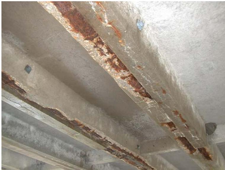
**FIGURE 4. Typical PCB Deterioration**
