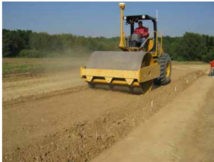
Figure 15. Caterpillar CS-533 vibratory smooth drum roller
