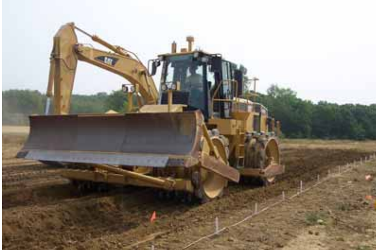
Figure 5. Compaction of test strip using 825G roller
