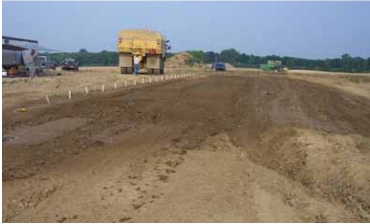
Figure 3. Moisture conditioning test strip
