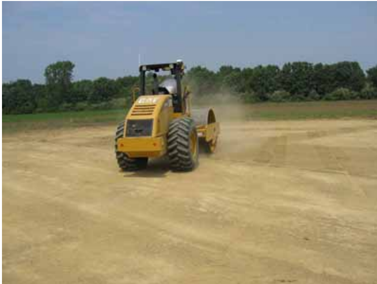
Figure 87. Preparation and compaction of spatial test area 1
