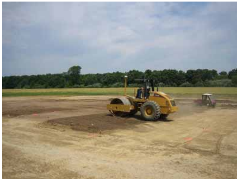
Figure 74. Compaction of Spatial 3
