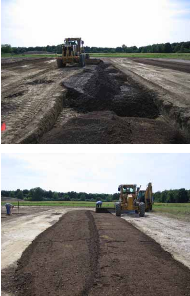
Figure 69. Placement of fill in Strip 2 excavation
