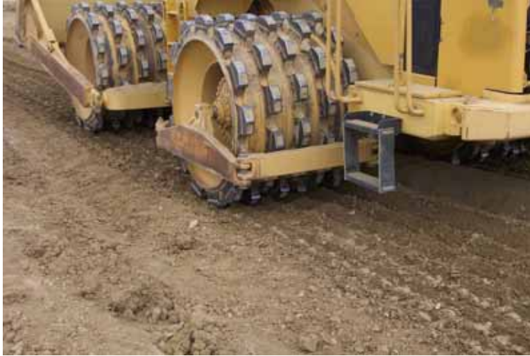
Figure 5. Compaction of test strip using 825G roller (cont.)
