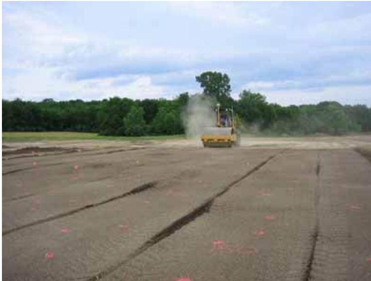
Figure 71. Compaction of Spatial 2
