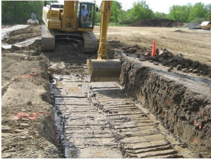
**Figure 66. Preparation of wet subgrade portion of TB 2**
