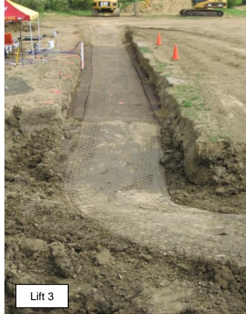
**Figure 45. Concrete base and lifts 1 to 3 of CA6-G material in TB 1**
