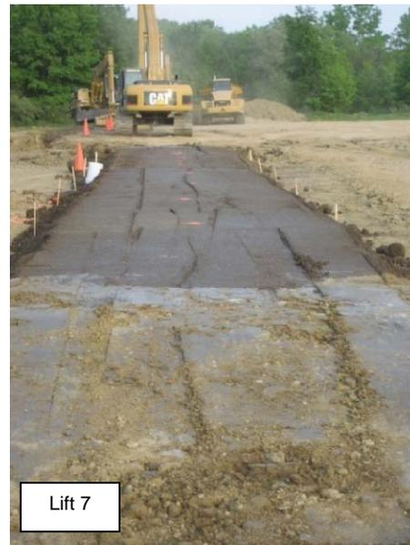
**Figure 68. Lifts 4 to 7 of CA6-G material placed in TB 2**
