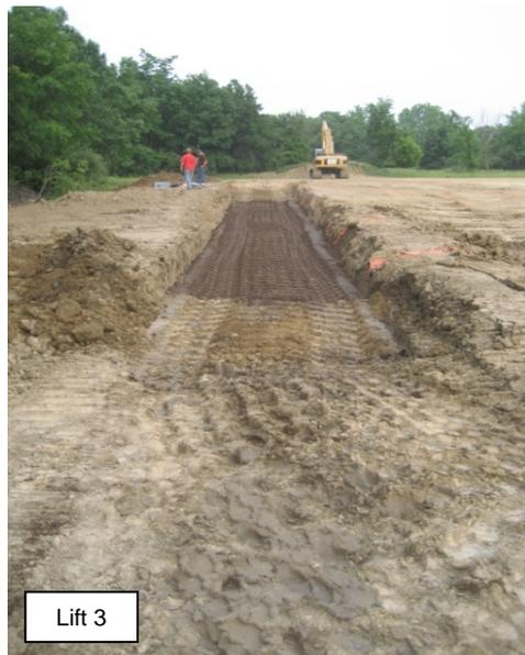
**Figure 84. Concrete and soft/wet subgrade base and lifts 1 to 3 of CA6-G material placed in TB 3**
