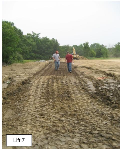
**Figure 85. Lifts 4 to 7 of CA6-G material placed in TB 3**
