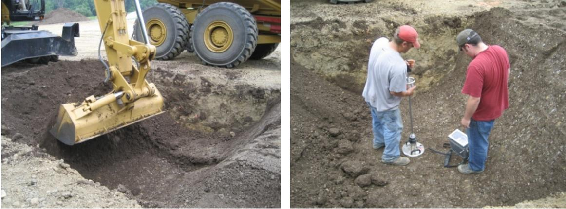
**Figure 86. Process of excavation to the top of each underlying lift to perform LWD testing**
