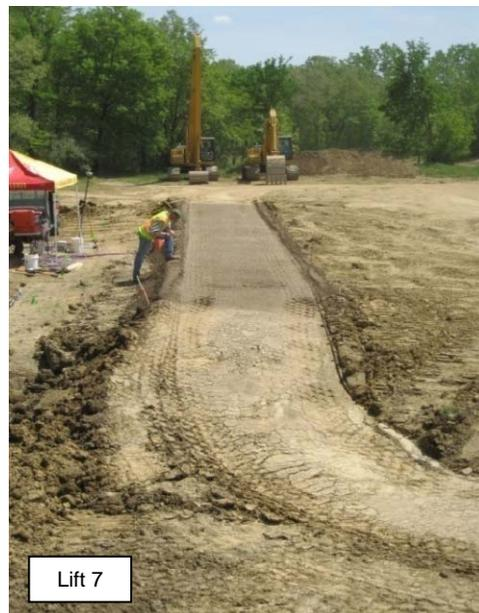
**Figure 46. Lifts 4 to 7 of CA6-G material placed in TB 1**
