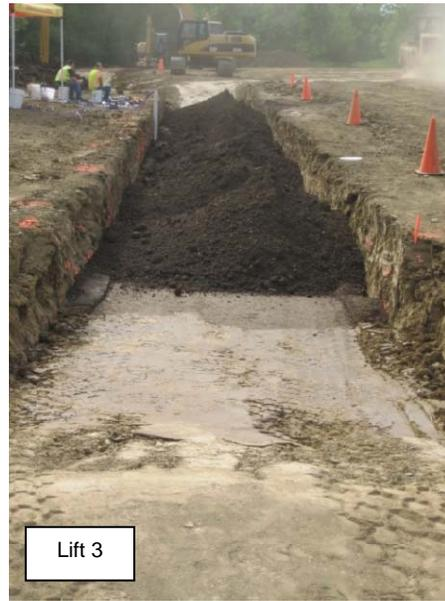
**Figure 67. Wet/dry subgrade and lifts 1 to 3 of CA6-G material placed in TB 2**
