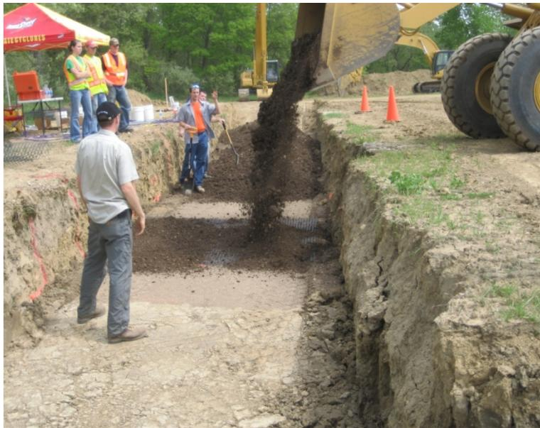
**Figure 47. Placement of biaxial Geogrid in TB 1**
