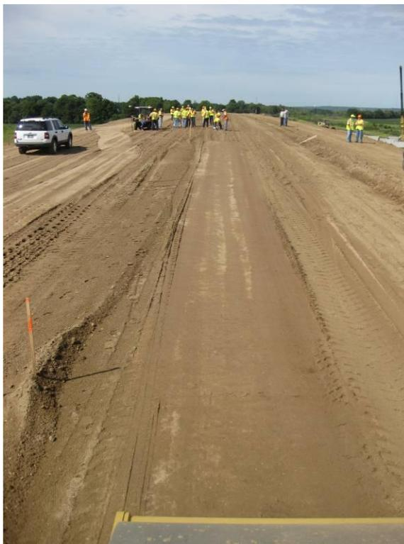
**Figure 10. TB1 granular embankment fill calibration test strips**
