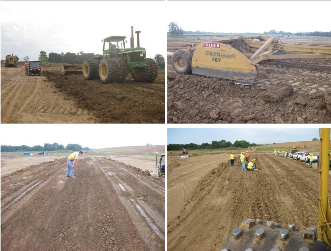
Figure 23. Construction of TB4 silty clay subgrade calibration test strips
