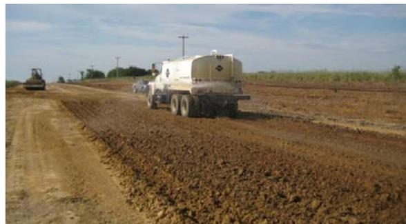
*Subgrade scarification using grader (top), disking (middle), and moisture conditioning (bottom)*
