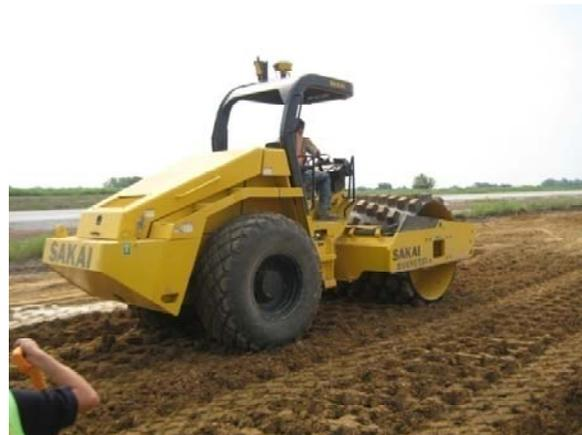
*Sakai SV610 padfoot roller used for compaction*
