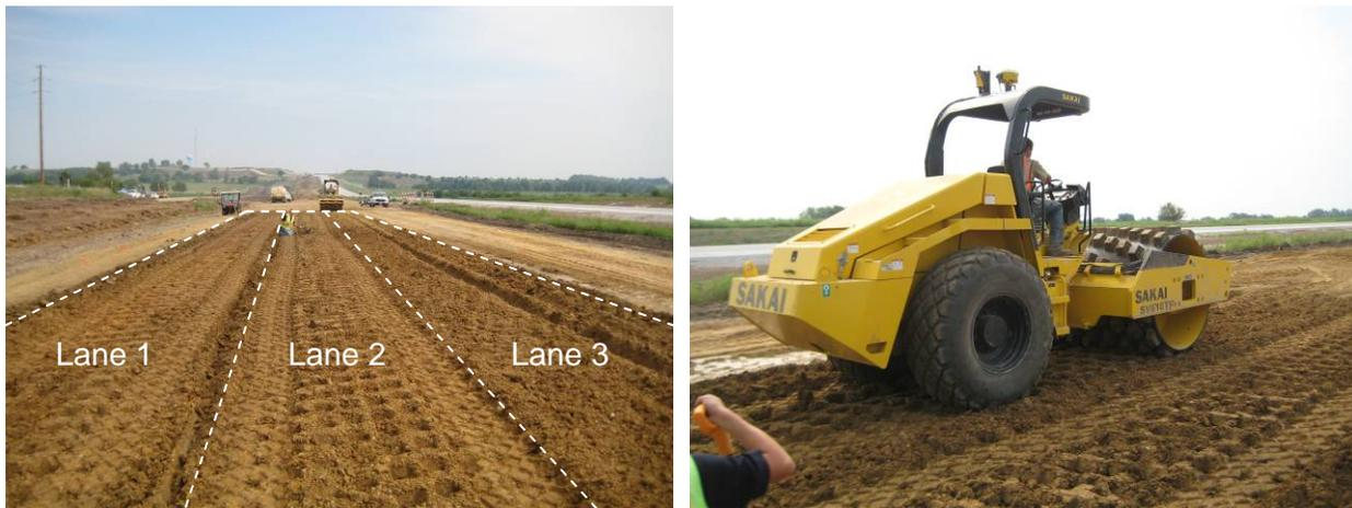
**Figure 25. Photographs showing construction and setup of lanes for compaction and testing on TB4 subgrade clay material**
