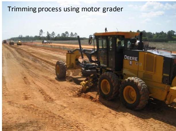
**Figure 38. Pictures showing construction process on TBs 5/6 treated subgrade**
