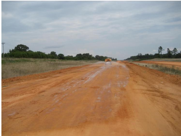
**Figure 31. TB4 compacted granular subgrade material**
