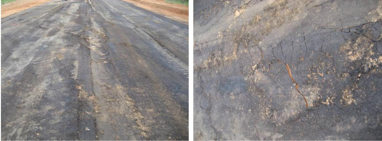
**Figure 18. Cracks observed on the treated base material following the Sakai vibratory roller pass – TB2**
