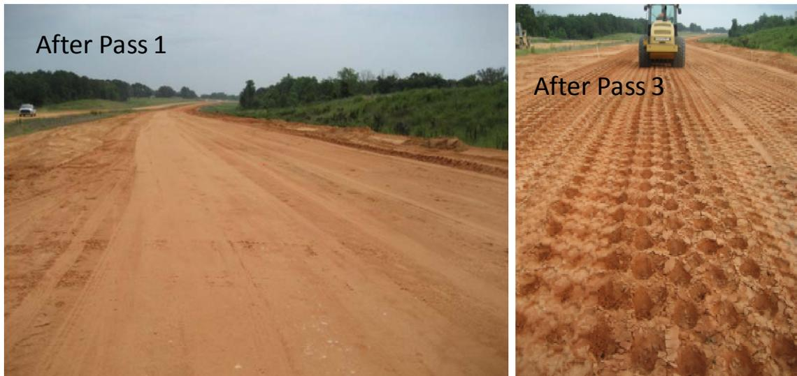
**Figure 10. TB1 granular base material after pass 1 with Sakai smooth drum roller (left) and pass 3 with Caterpillar padfoot roller (right)**
