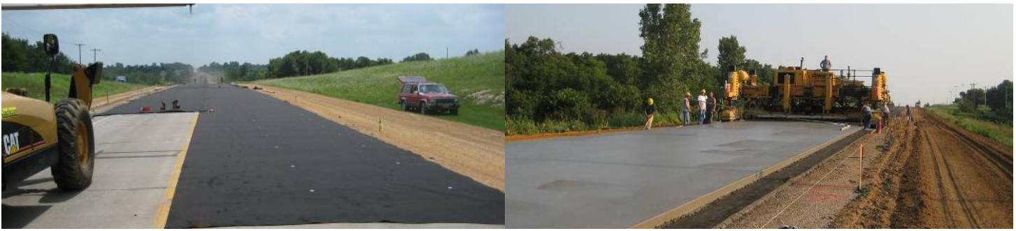
Figure 11. Construction of Unbonded Overlay with Nonwoven Geotextile Interlayer.
