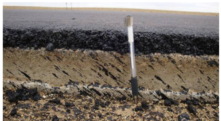
Figure 13. Asphalt Separation Layer.
