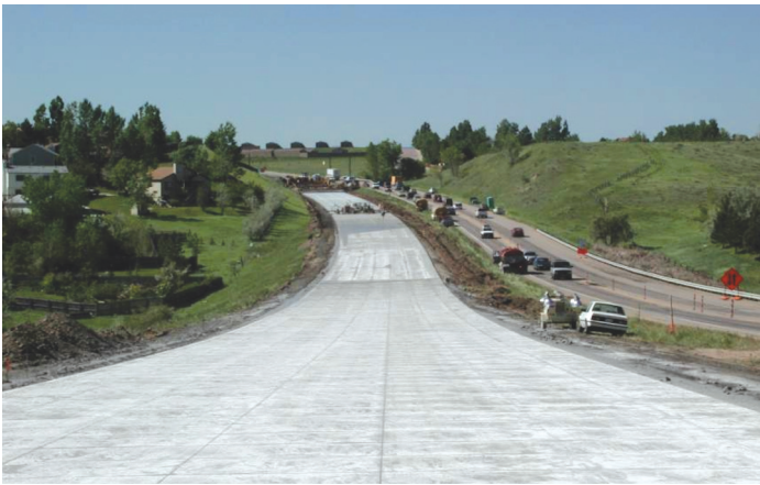
Figure 8. Bonded Concrete Overlay of Asphalt Pavement.
